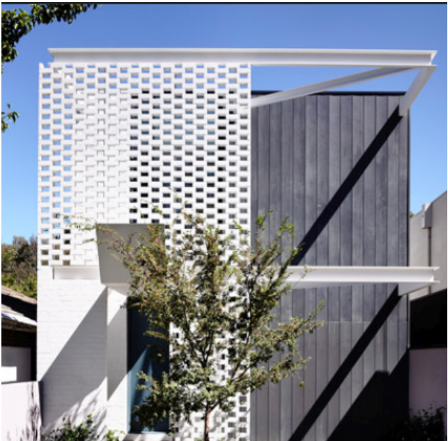
Figure 2-72 Privacy screens are integrated into the facade and provide part of the architectural expression
