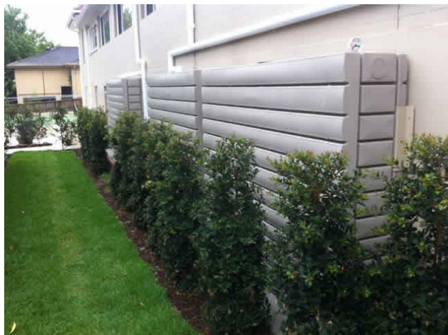
Figure 2-116 Integrate rainwater tanks into the landscape
