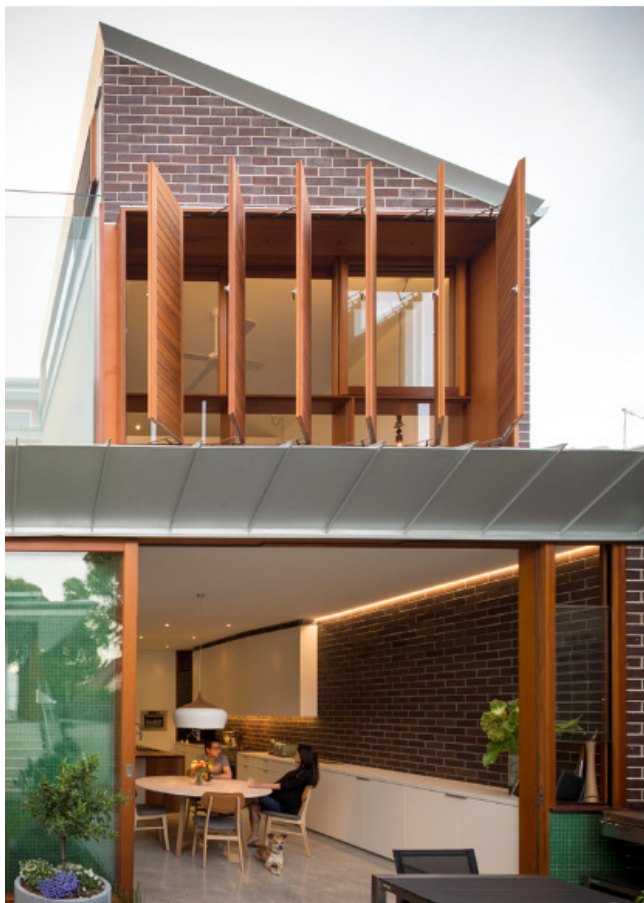
Figure 2-109 Adjustable screens allow control of sunlight.
