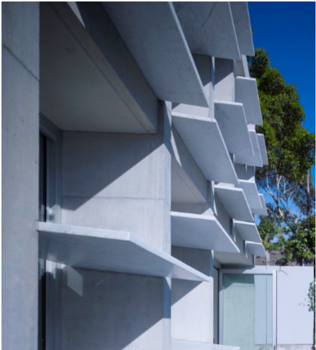
Figure 2-107 Light shelves can reflect sunlight deeper into rooms and provide shade from summer sun.
