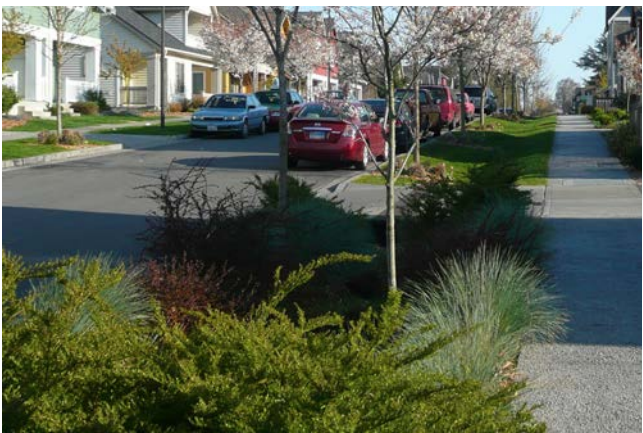
Figure 2-111 Swales can be attractive, filter and collect the stormwater
