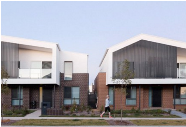
Figure 2-98 Use of screens provides privacy and suncreening to balconies.
